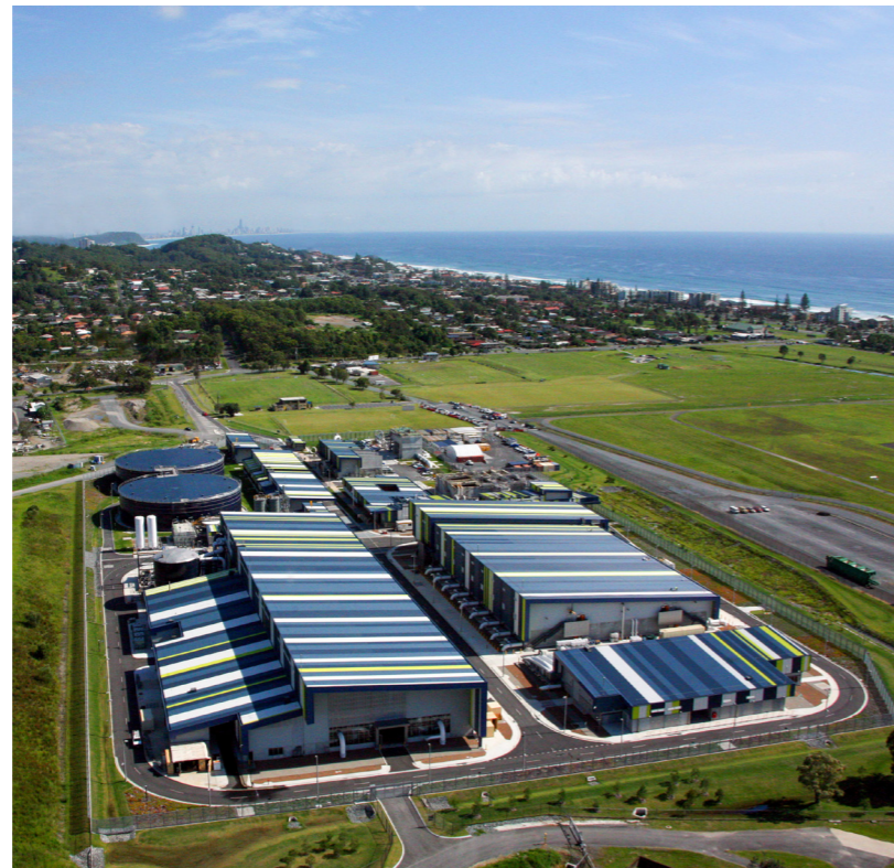
Gold Coast Desalination Plant, image from Seqwater.
